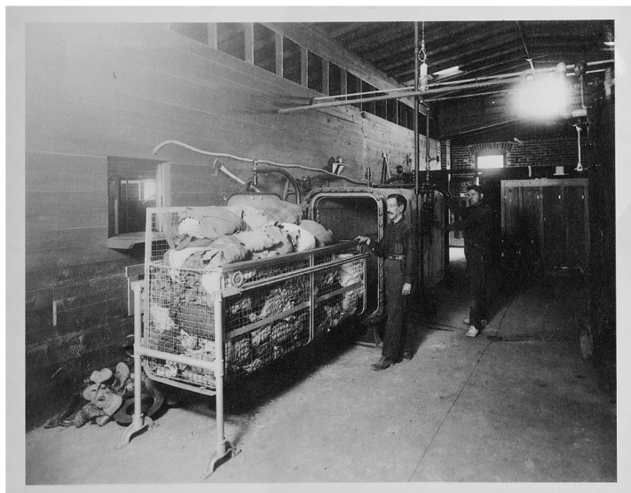
Steam dryer for sterilizing clothing at the Santa Fe Bridge, 1917. (U.S. Public Health Service, National Archives)
